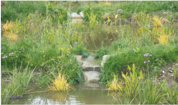
Figure 4.5 Example demonstrating how the wetland cells can be designed to minimise the risk of short-cutting
