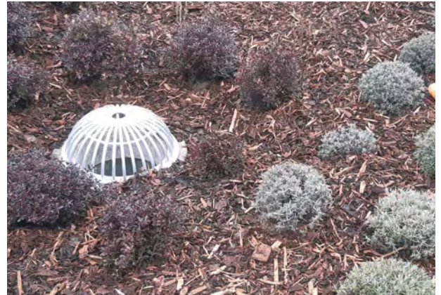
Domed grille less risk of blocking than a flat grille but not suitable for high flows
