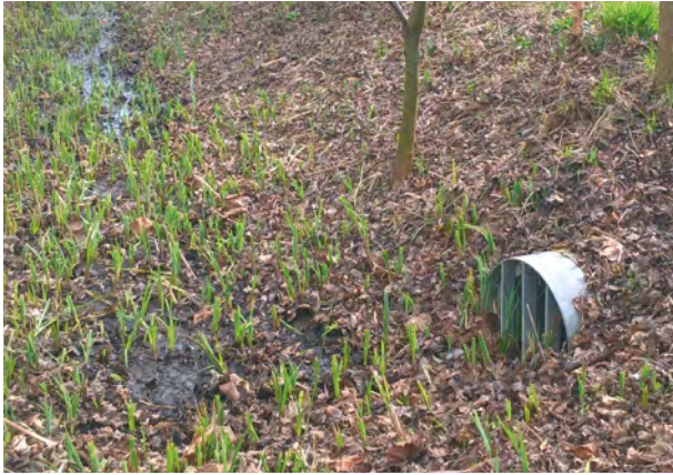
Vertical grille same size as outlet pipe – requires regular maintenance, for low flows only unless used in combination with an overflow
