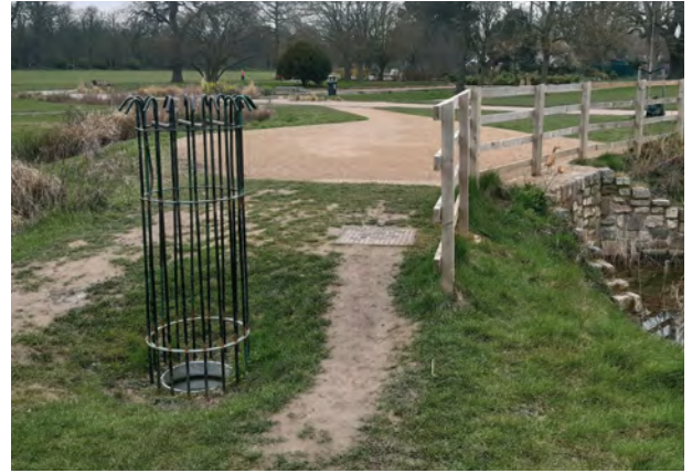
Tall circular grille provides relatively high flow capacity with low risk of blockage
