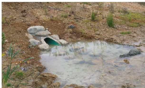
Example of piped crossing between two cells
